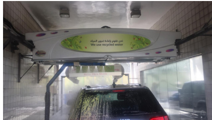
Exhibit 29: A. Water recycling car wash system in Emirates National Oil Company's retail stations B. Car wash system water meter
